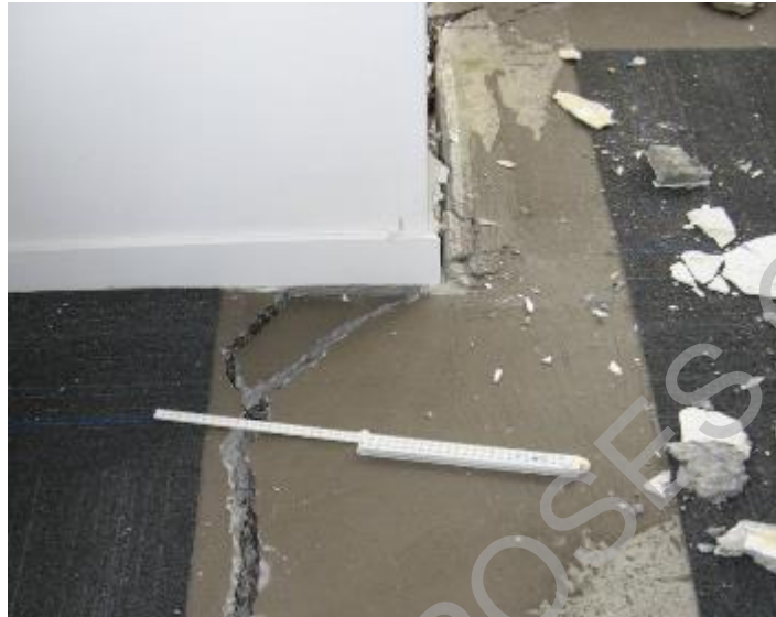
Figure C5.37: Observed separation between floor and supporting beam due to beam elongation in 2011 Canterbury earthquakes (Bull)
